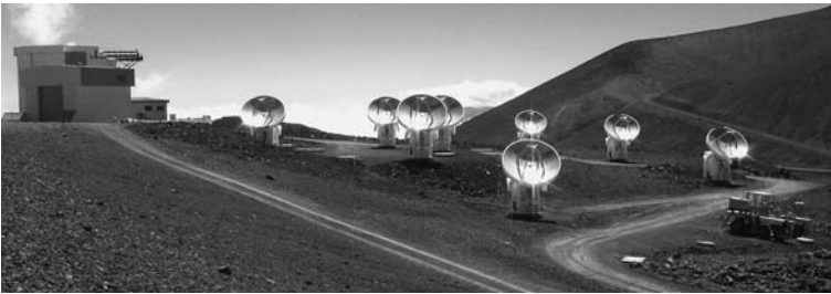
Fig. 9.9 The Sub Millimeter Array (SMA) consists of eight 6-m antennas that are designed to operate to 0.3 mm, with a total geometric collecting area is 226 m 2 . The SMA is located on Mauna Kea, at an altitude of 4.1 km. It was built and is operated by the Harvard-Smithsonian Center for Astrophysics (CfA) and the Academia Sinica Institute for Astronomy & Astrophysics (ASIAA), Taiwan (photo courtesy of N. Patel, CfA.)
