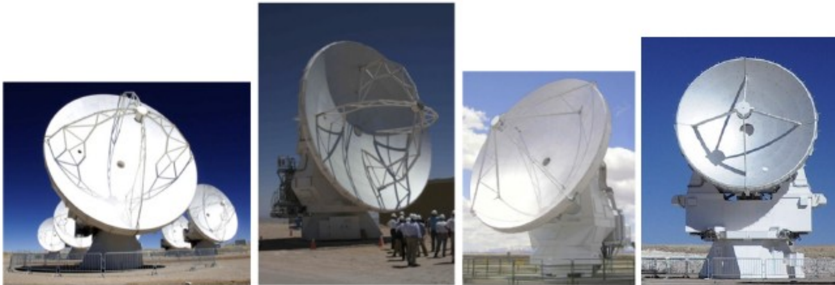
Figure A.1: The four different ALMA Antenna designs: Vertex 12 m, MELCO 12 m, AEM 12 m, and MELCO 7 m (from left to right).
